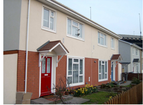
BISF Houses, Shirehampton — £200,000 — Insulated render with options of spar dash, brick effect and through-coloured acrylic render finishes.
