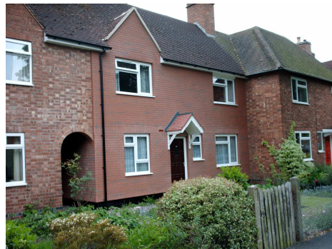
St Laurence Avenue, Warwick — £200,000 — Insulated brick effect render, fascias, soffits with associated building and plumbing works.
