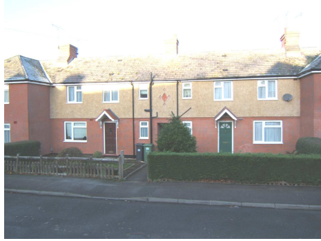
Hyde Road, Kenilworth—£425,000 —Insulated brick effect, through-coloured render, fascias, soffits with associated building and plumbing works.
